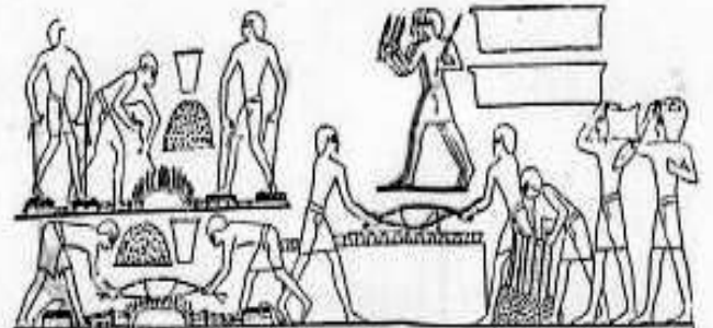
FIGURE 36j—Casting a bronze door. The bronze is melted in a crucible on an open fire with forced draught from four feet below. Best pieces of wood serve to lift the crucible to the mould in the centre, which has a series of spigets. One of the men on the right carries an ox-hide ingot. From a tomb at Thebes. c 1500 B.C.
